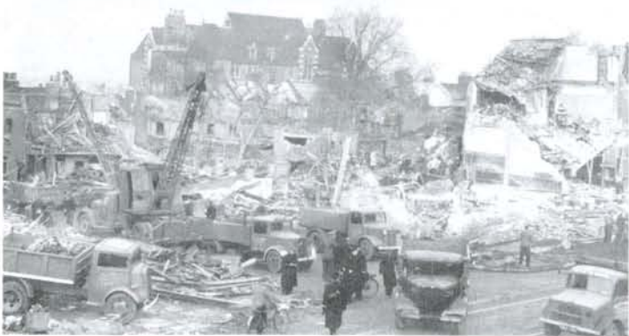
V-2 Damage (160 people were killed in this attack.)
